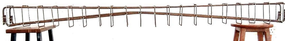
Figure 3.9: Front view reinforcement cage for Specimen 4.
