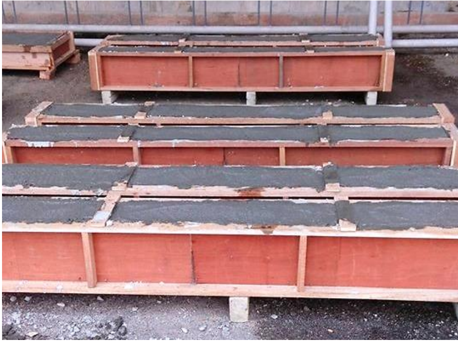
Figure 2: Casting of reinforced concrete beam.
