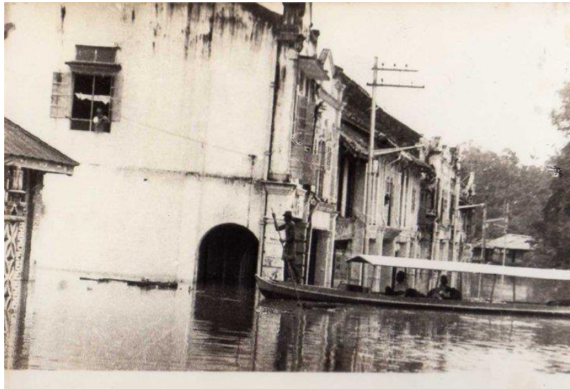
Figure 2.5 Flood in Kuala Lipis 1971 (courtesy: Nan Zul, Dec 2013)
