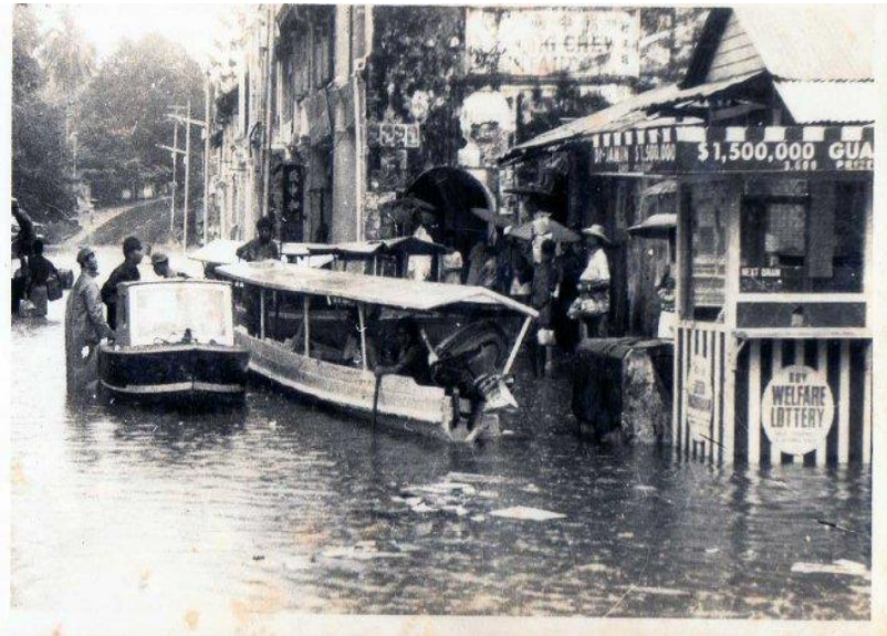
Figure 2.6 Flood at Jalan Jelai year 1971 (courtesy: Nan Zul, Dec 2013)
