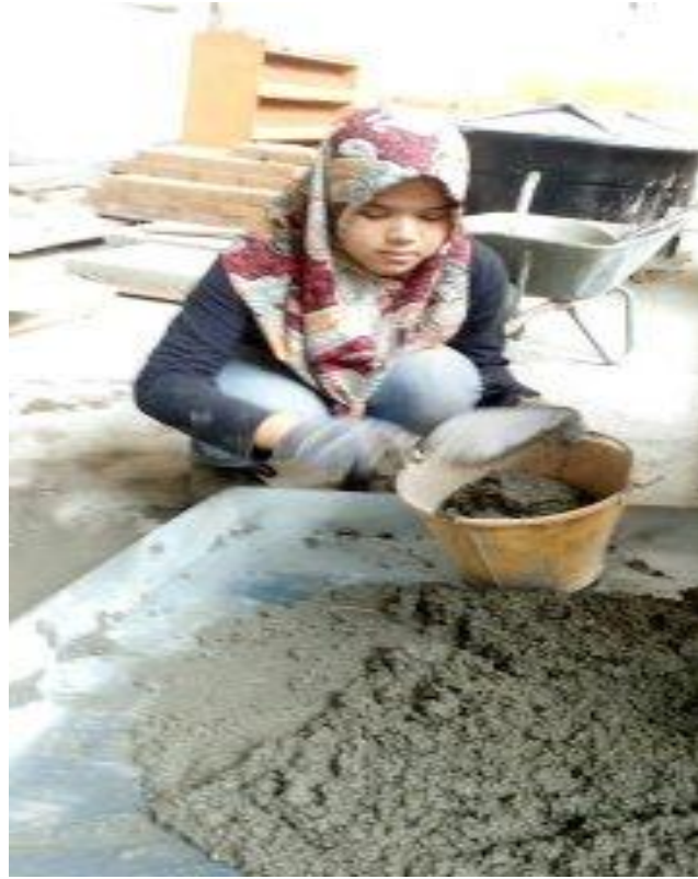
Figure 3.8: Scope the concrete into the bucket
