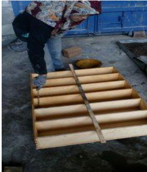
Figure 3.7: Oiling the formwork using hydraulic oil
