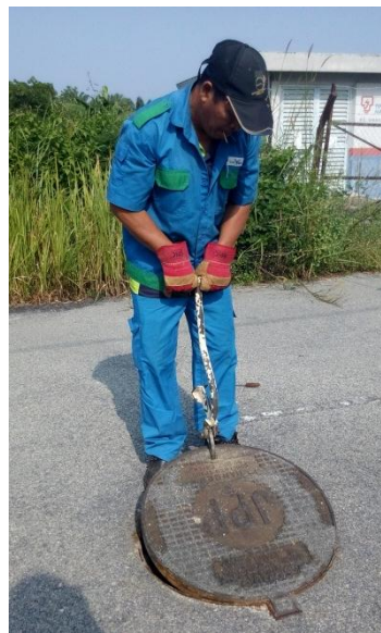
Figure 3.10: Staff from IWK using manhole opener to open manhole
