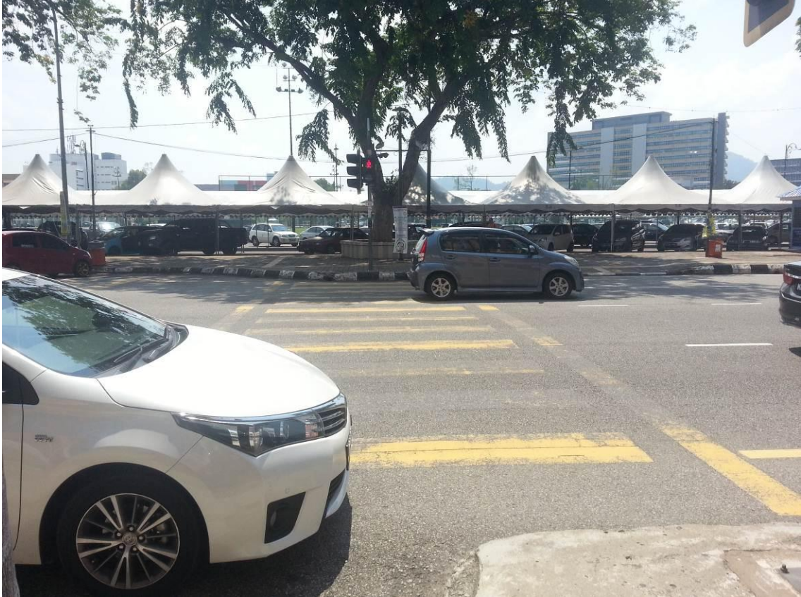
Figure 3.2: Signalized crossing at Jalan Mahkota
