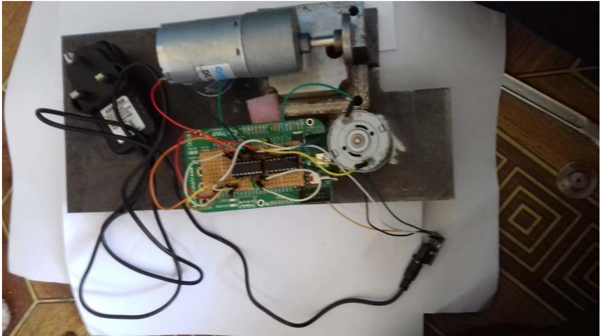
Figure 4.2: The electrical circuits and its position on the mechanical parts of the project
