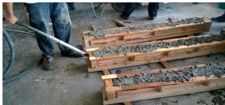
**Figure 3.16:** Fresh concrete was vibrated using a vibrator
