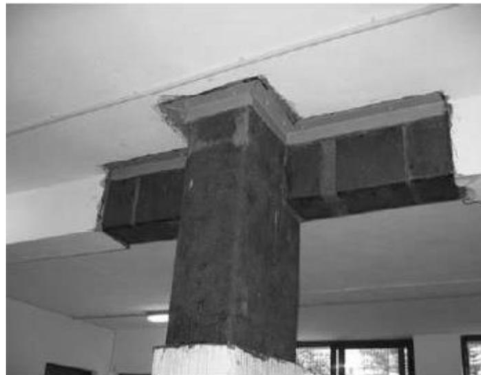
**Figure 2.13:** Strengthening of RC beams
