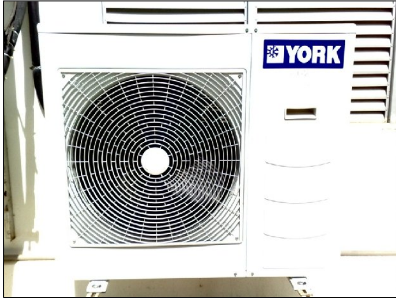
Figure 4.2: Heat blow from one condensing unit will be use to dry clothes
