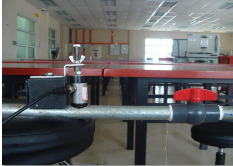
Figure 3.4: Suitable locations for sensor placement for ball valve classifying test.
