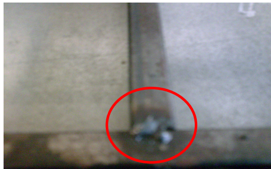
Figure 4.9: The weld that not been grinded
