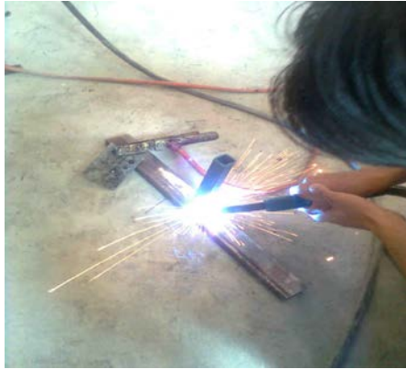
Figure 3.3: Welding process using MIG welding
