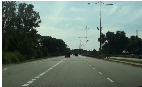
Fig. 2. Current Condition of Road between Batu Enam and Pekan
