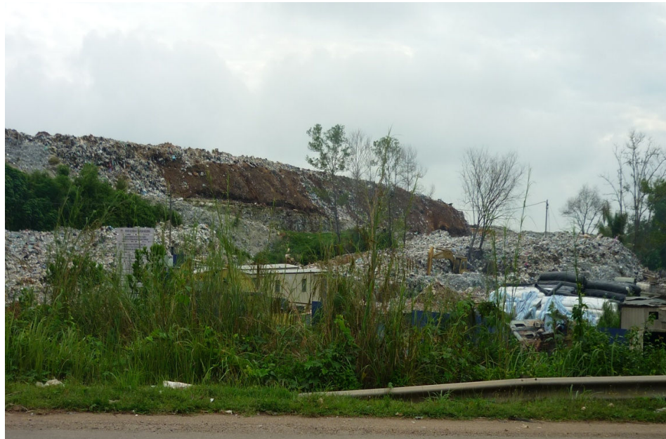
Figure 1.2: Newly closed landfill in Ulu Tualang
