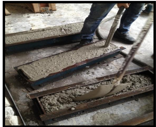
Concrete poured & vibrated
