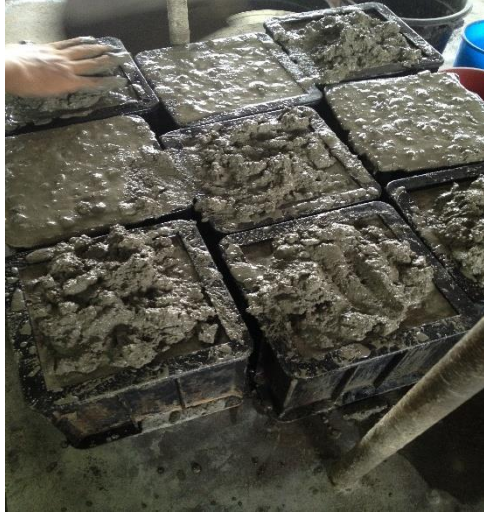
Filled & vibrated the concrete
