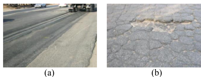
Figure 2. (a) Rutting; (b) Fatigue cracking
