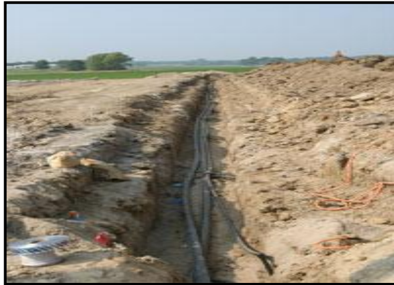
Figure 2.7: Ground Heat Exchanger
