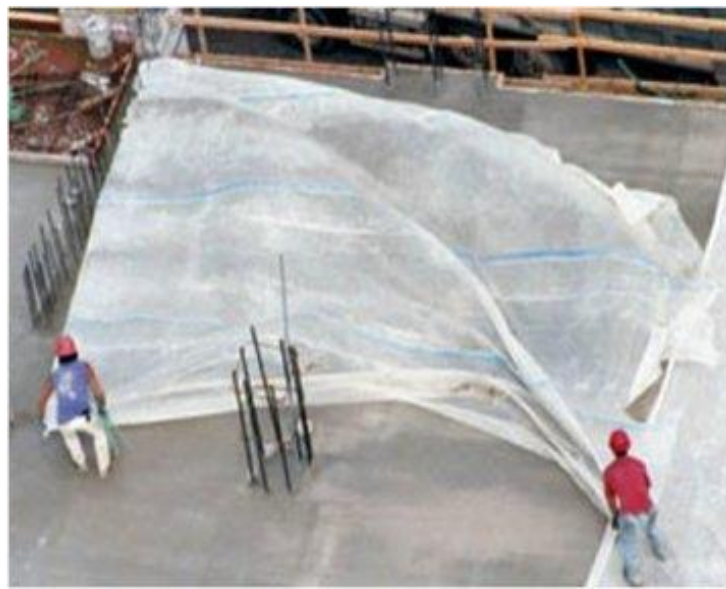
Figure 2.5: Plastic sheet concrete curing method
