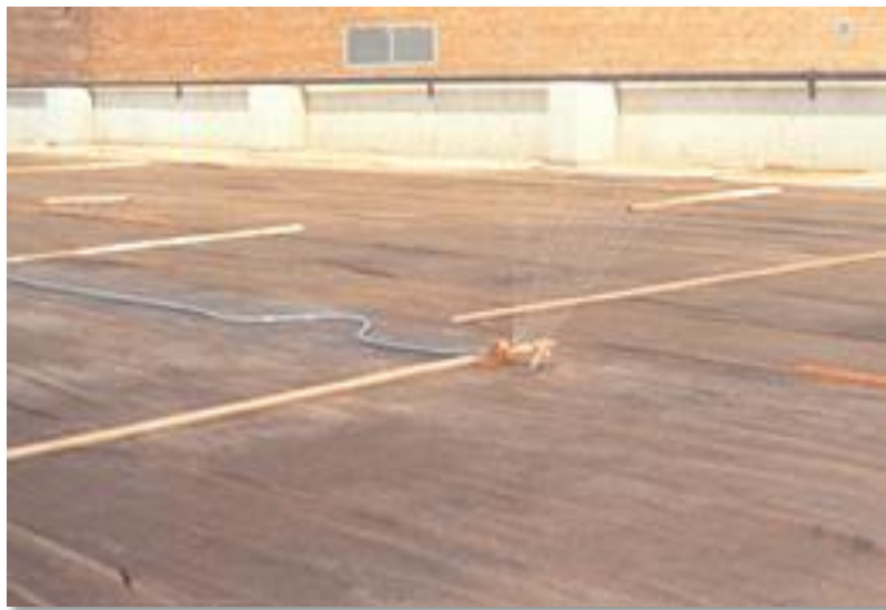
Figure 2.8: Sprinkling curing method
