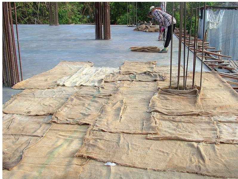
Figure 2.4: Wet covering concrete curing method
