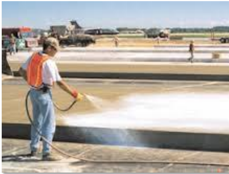
Figure 2.7: Membrane-forming curing compound method
