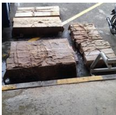
Curing by using wet gunny sacks
