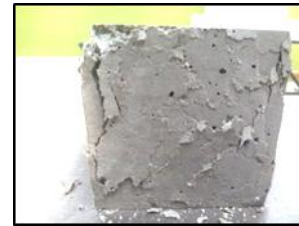
(e) The crack patterns cube sample of 10% for 28 days
