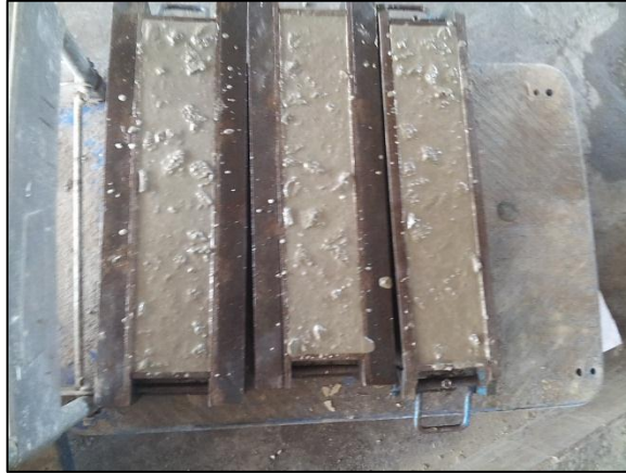
Figure 3.17: Casting concrete for beams already done
