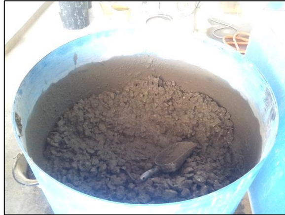
Figure 3.13: The concrete has already done in mixing
