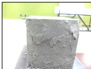
(b) The crack patterns cube sample of 2.5% for 7 days
