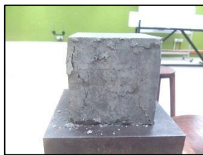
(b) The crack patterns cube sample of 2.5% for 14 days
