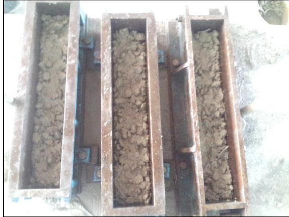
Figure 3.15: The process of placing concrete into the cylinder and beam moulds
