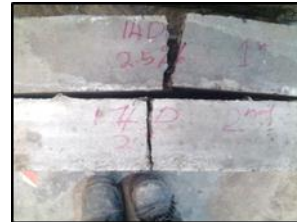
(b) The crack pattern beam samples of 2.5% for 14 days
