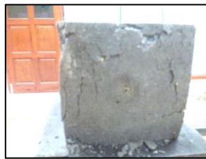
(a) The crack pattern of cube sample of 0% for 28 days
