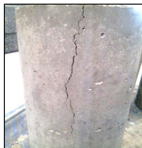
(b) The crack pattern cylinder samples of 2.5% for 14 days
