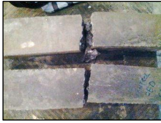
(a) The crack pattern beam samples of 0% for 28 days
