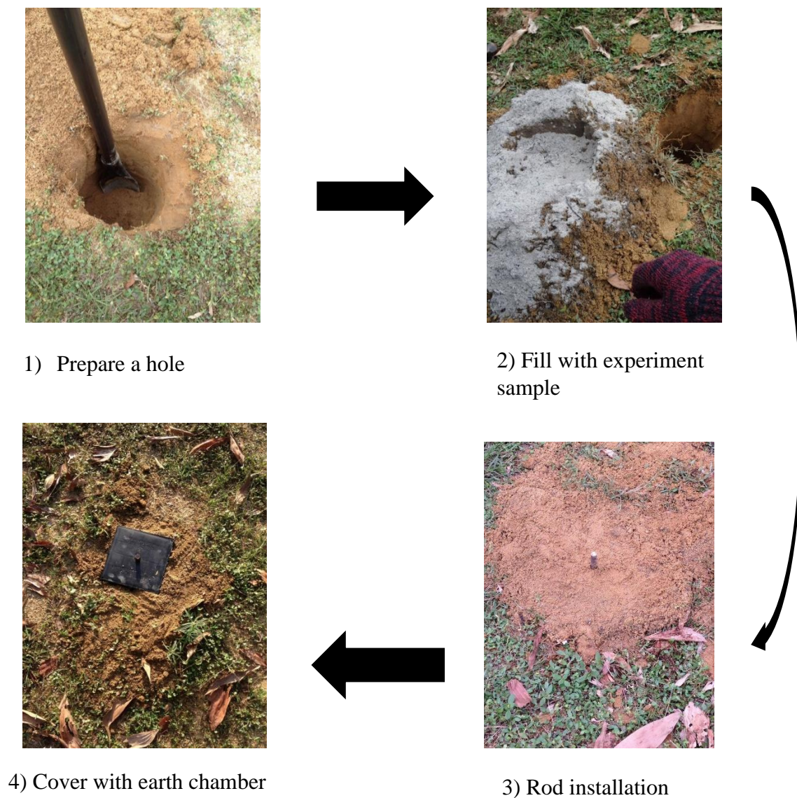
Figure 3.6: Installation Process of Grounding System
