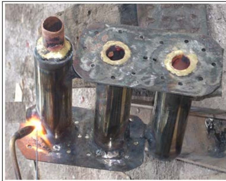
Figure 4.9: Welding on steel plate and stainless steel pipe
