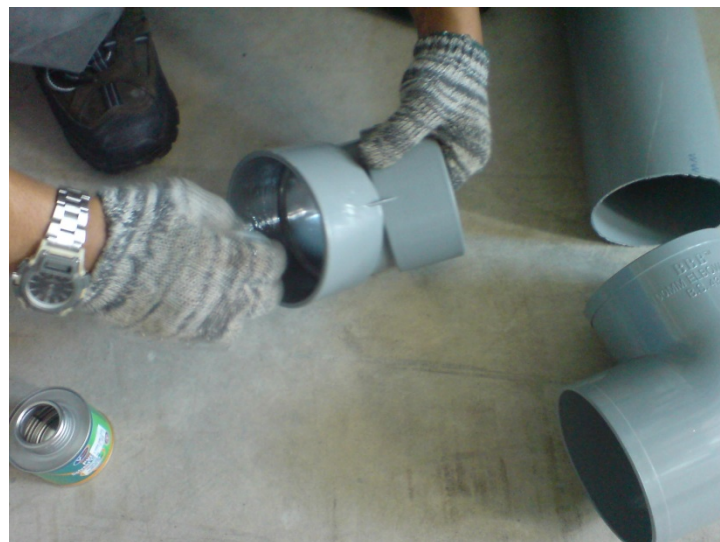
Figure 3.9: PVC elbow and glue
