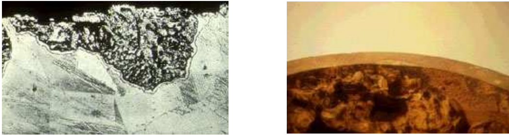
Figure 2.5: The brass on the left dezincified leaving a porous copper plug on the surface. The gray cast iron water pipe shown on the right photo has graphitized and left graphitic surface plugs which can be seen on the cut surface [1] (Source: NASA Corrosion Technology Laboratory)
