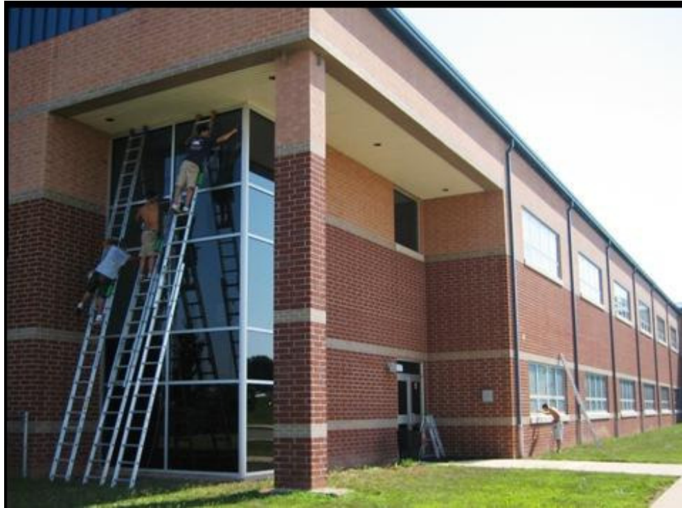
Figure 2.7: Cleaning method using ladder
