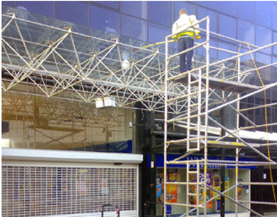
Figure 2.6: Cleaning method using scaffold
