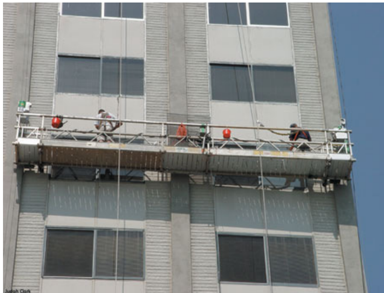
Figure 2.2: Cleaning method using gondola
