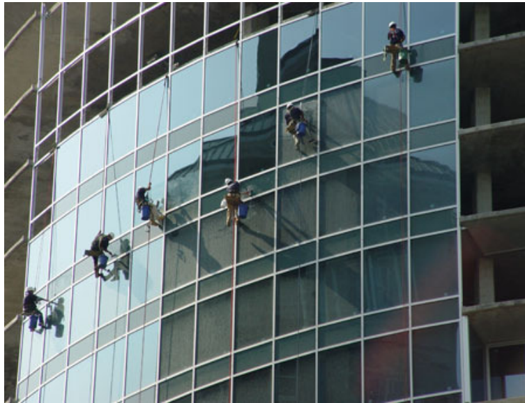
Figure 2.1: Cleaning method using abseiling technique
