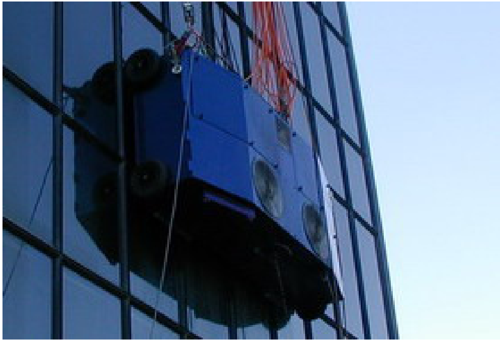
Figure 2.8: Cleaning method using customized window cleaning machine
