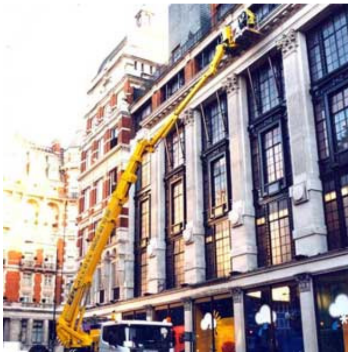
Figure 2.5: Cleaning method using working platform
