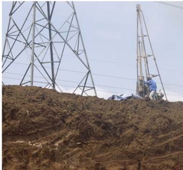
Figure-1. Drilling rig operated on top of the slope.
