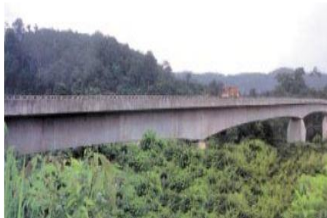
Figure 1.2: Concrete Bridge, Sultan Abdullah Bridge, Jerantut Pahang
