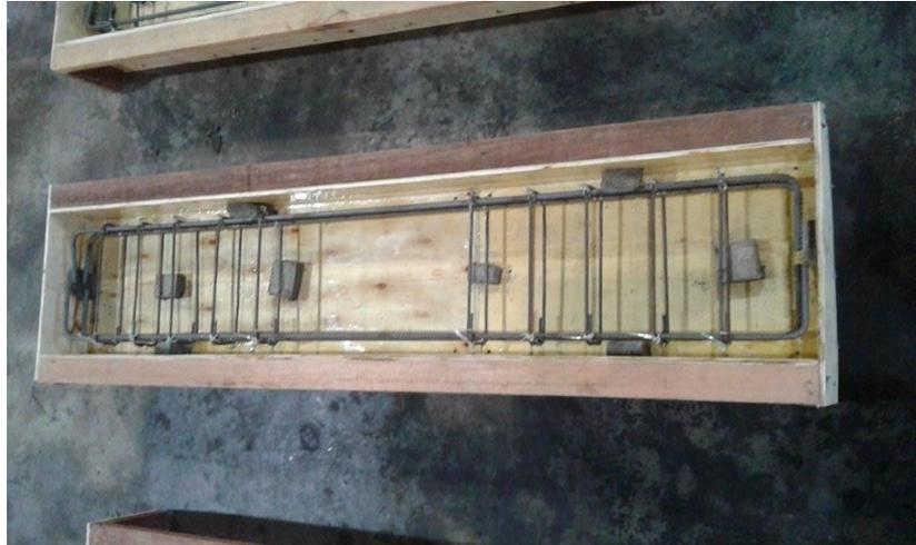
**Figure 3.11:** Formwork for reinforced concrete solid beams
