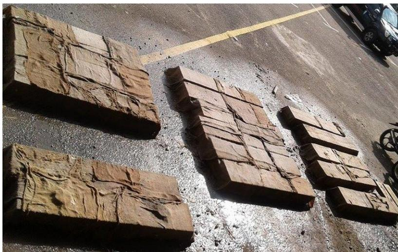
**Figure 3.22:** Beam curing process
