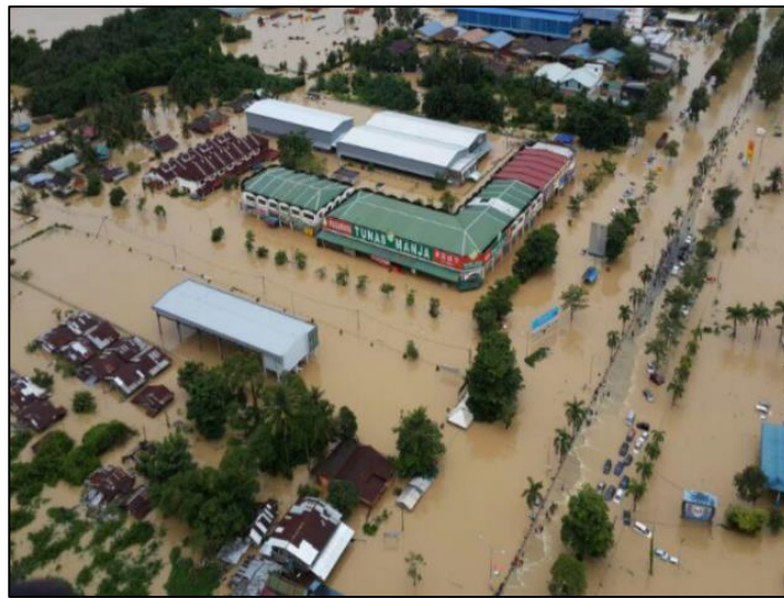
Figure 1.5: Flood Event 2013 at Sungai Isap
