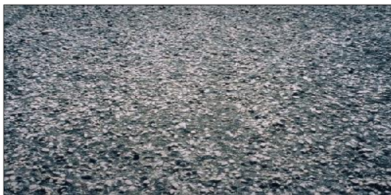
Figure 2.5 Polished Aggregate Problem
