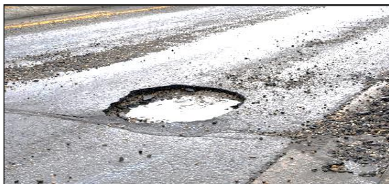
Figure 2.3 Pothole damage
