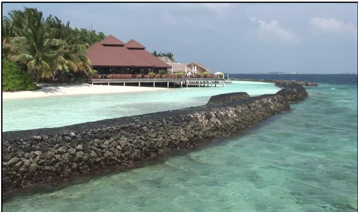
Figure 4.11 Wave Breaker at Maldives
