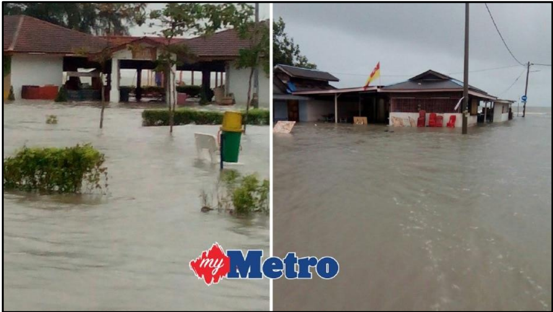
Figure 2.16 Seawater Overflow at Pantai Kelanang, Banting, Malaysia
