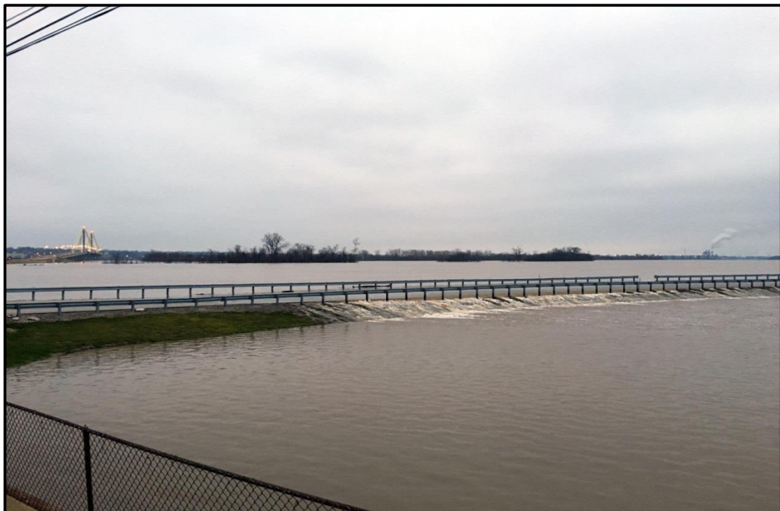
Figure 2.4 Overtopping Along the Riverland Way, Australia
