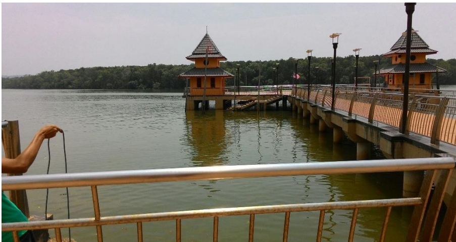
Figure F2: Station 2 view
