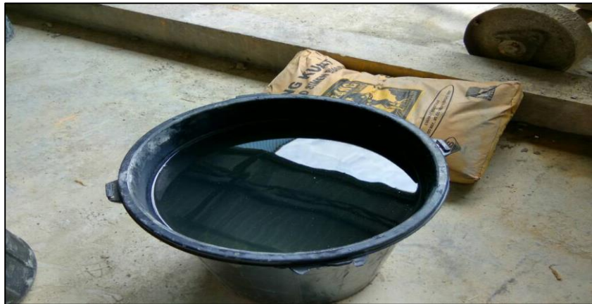
Figure 3.7: Water Use to Mix the Concrete
