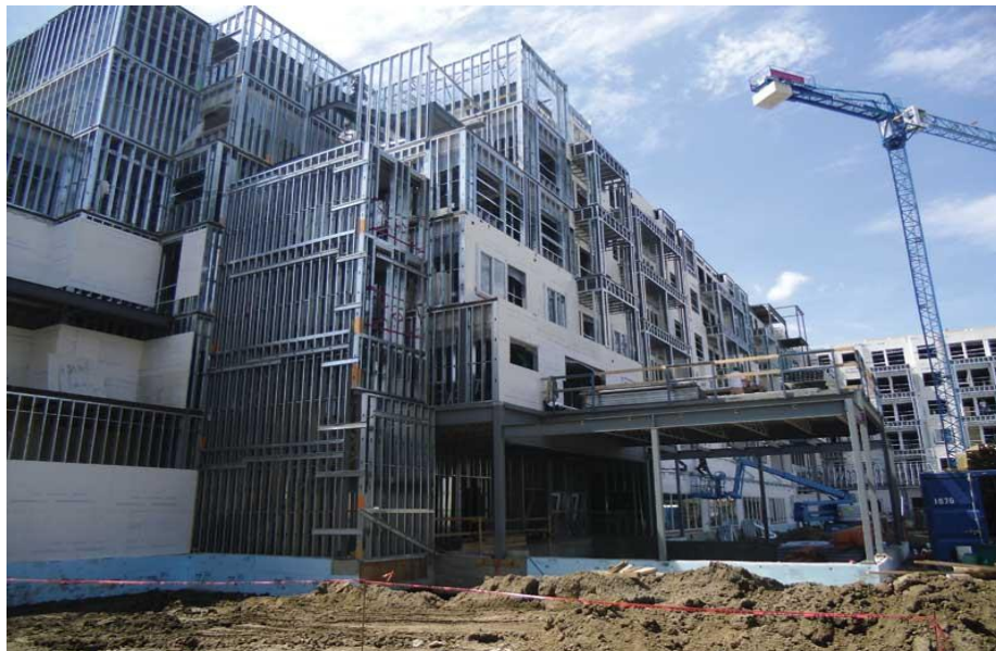
Figure 1.3 Cold-formed steel framing
