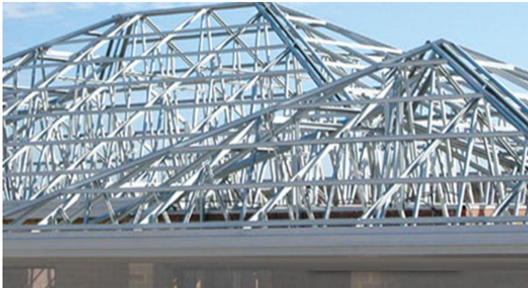
Figure 2.2 Roof system using cold-formed
