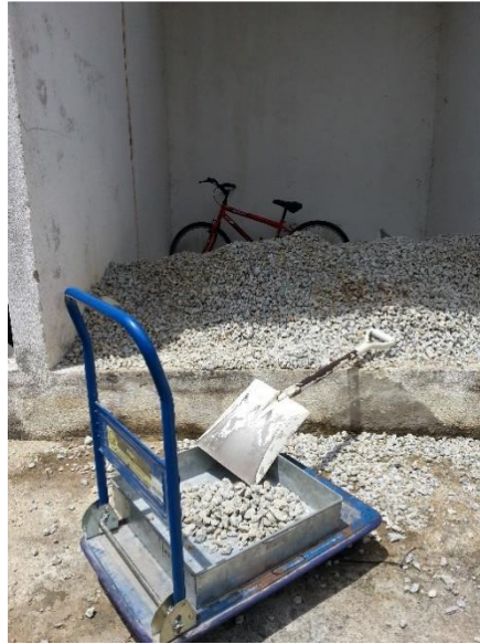
Figure 3.3: Delivering aggregates from store
