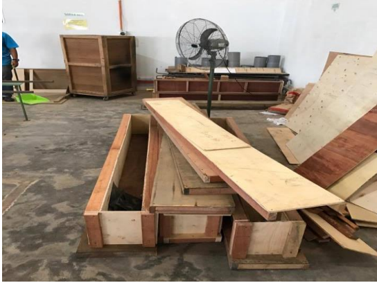
Formwork preparation
