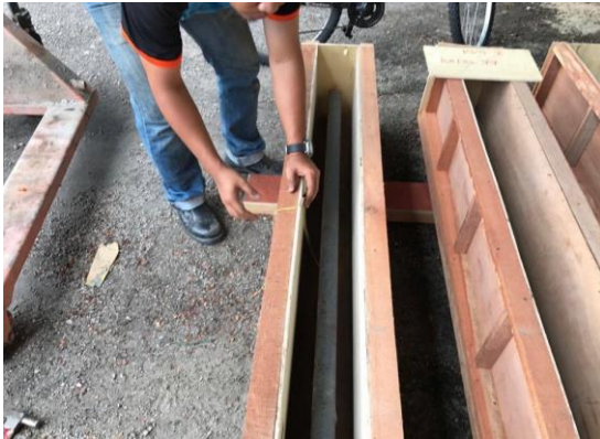
Steel I-Beam cast into the formwork
