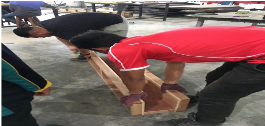
Figure 3.6 Formwork for beam
