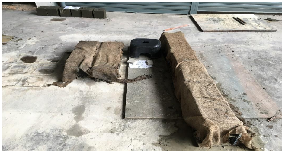
Figure 3.9 Curing process using wet covering
