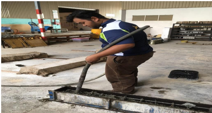
Figure 3.8 Compaction work
