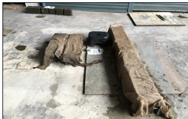
Figure 3-17: Wet Burlap Coverings
