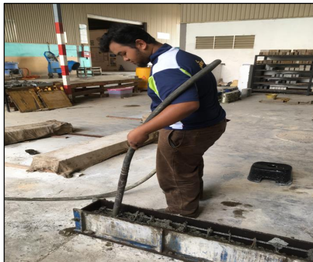
Figure 3-15: Compaction Process
