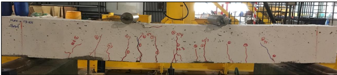
Figure 4-15: Cracking Pattern of RCA-SF1% beam
