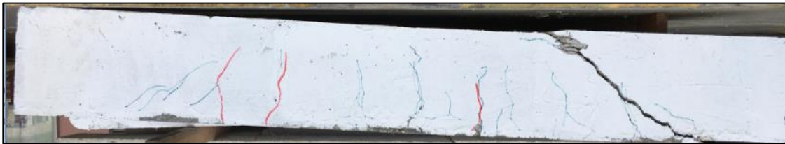
Figure 4-14: Cracking Pattern of RCA beam
