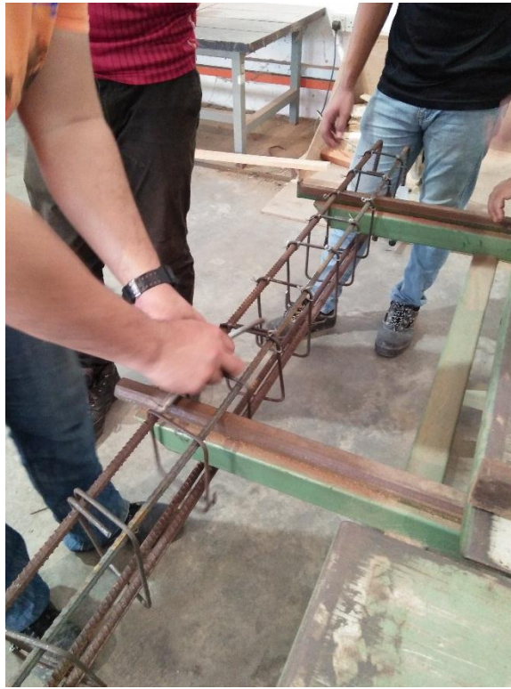
Figure 3.7: Preparation of steel reinforcement
