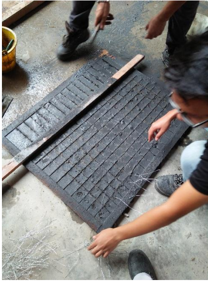
Figure 3.8: The making of concrete cover
