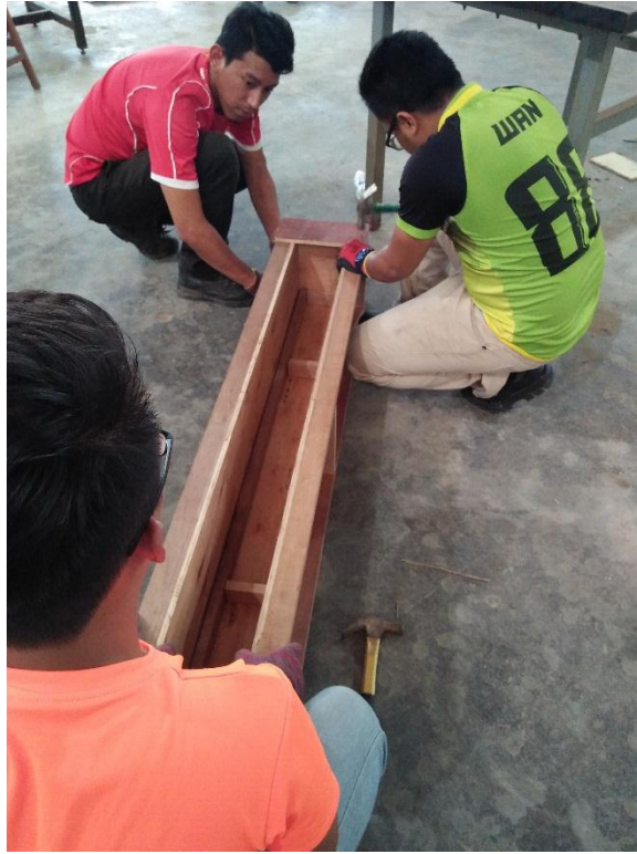
Figure 3.6: Preparation of formwork
