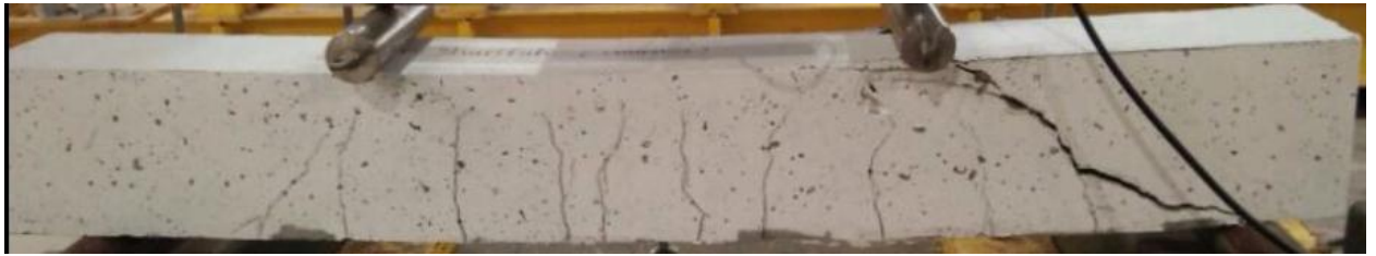
Figure 4.11 : Cracking pattern for controlled beam(NCA)
