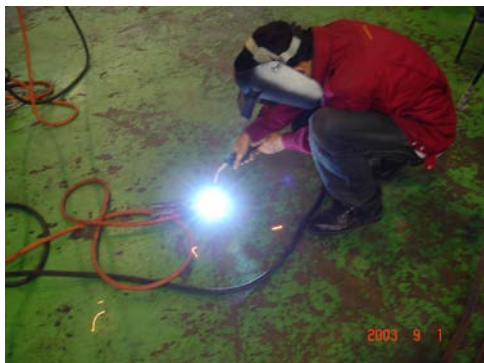
Figure 3.15: Joining process by using MIG weld
