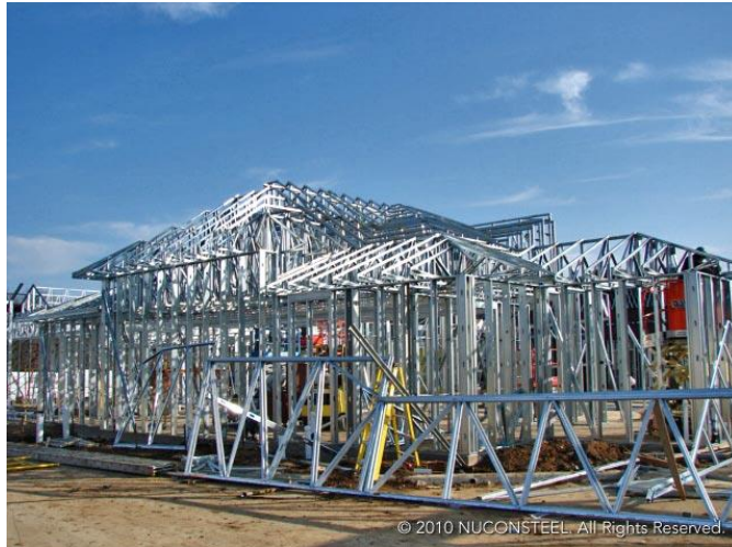
Figure 1.2: Residential area using cold-formed steel
