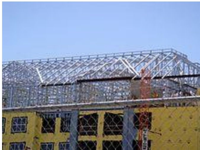
Figure 1.1: Roof truss using cold-formed steel
