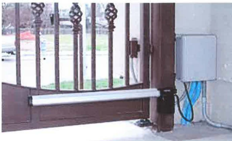
Figure 2.3: Picture of mechanical ram arm
