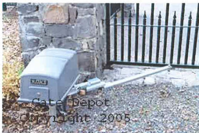
Figure 2.1: Picture of bottom mounted swing arm
