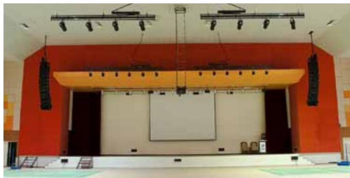
Audio System : Line array speaker, stage fill speaker, front fill speaker, monitor speaker and sub woofer
