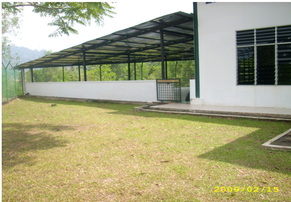
Figure 4.11: Location of AHU room at North-West side
