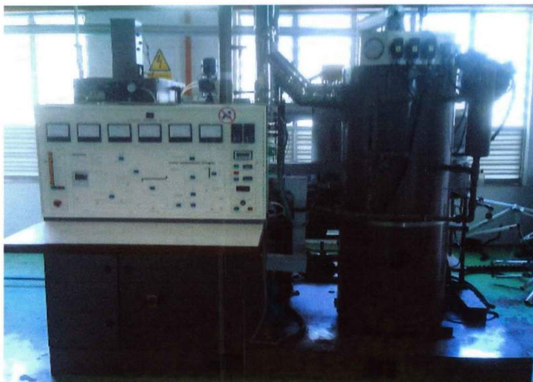
Figure 2.5: Cussons steam power plant
