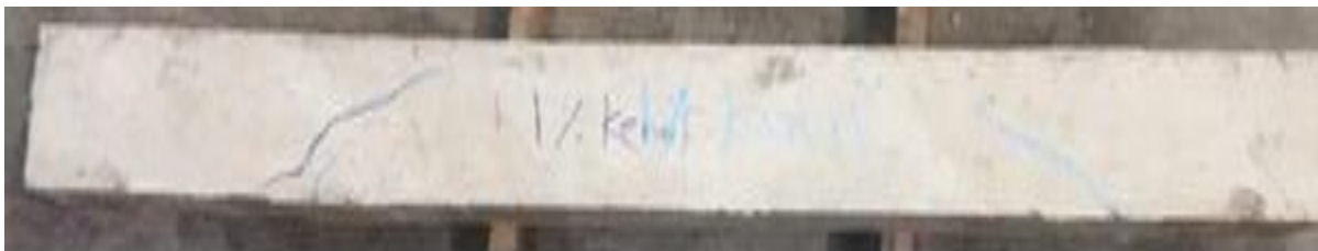
Figure 4.11: Failure mode and crack pattern of 1% kenaf fiber beam
