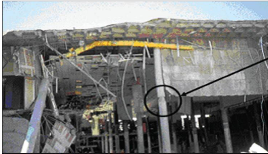
Figure 2.14: Building collapse due to punching of the flat slab.
