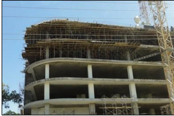
Figure 1.2 : Flat Slab in construction building
