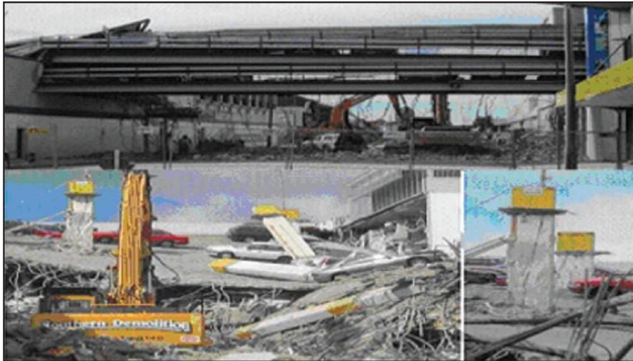
Figure 2.13: Punching Shear Failure in flat slab.
