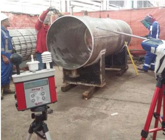
QUESTemp°34 Thermal Environment Monitor and Anemometer were placed near the welding area
