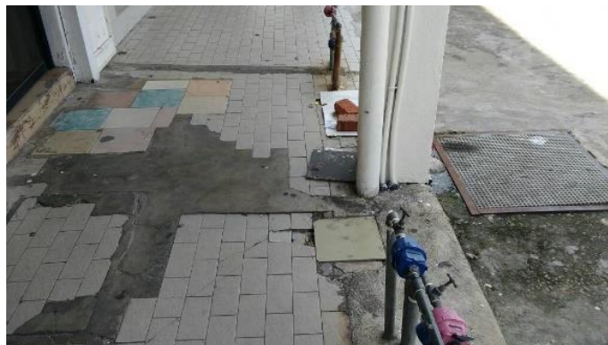
Figure 4.6.4.f: Improper pavement
