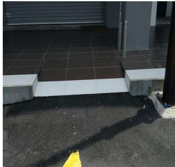
Figure 4.8.2. b: Kerb ramp
