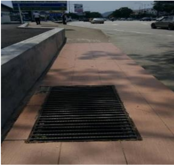
Figure 4.6.3.a: Walkway that connecting Zone 2 and Zone 3
