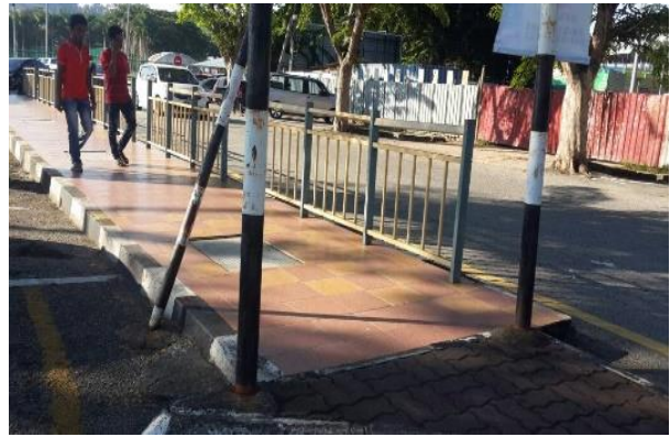
Figure 4.6.1.b: Tile type pavement
