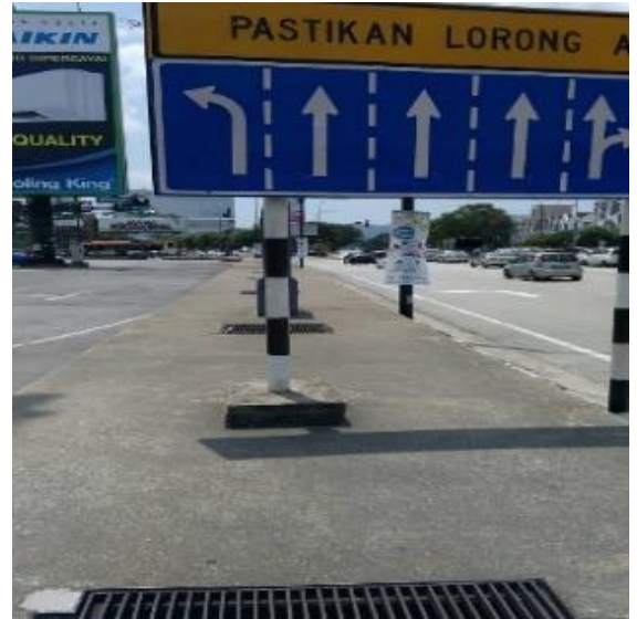
Figure 4.6.3.b: Signboard in the middle of the walkway
