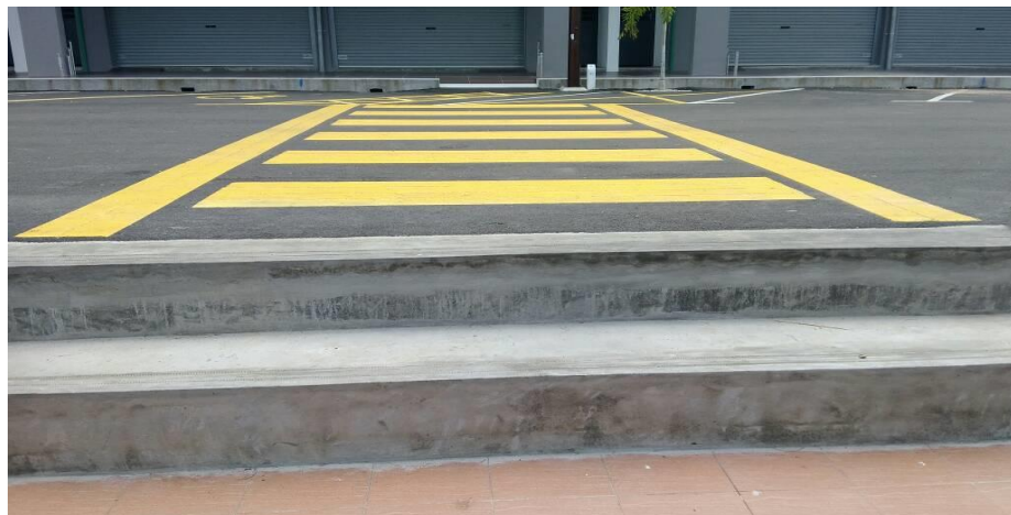
Figure 4.10.2. b: Zebra crossing between zone 2 and zone 3 but it is improper because no ramp provided
