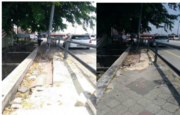
Figure 4.6.1.c: Improper pavement
