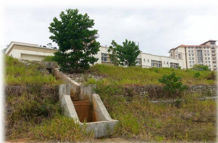
Figure 3.9 Front View of the Building (Toe of Slope)
