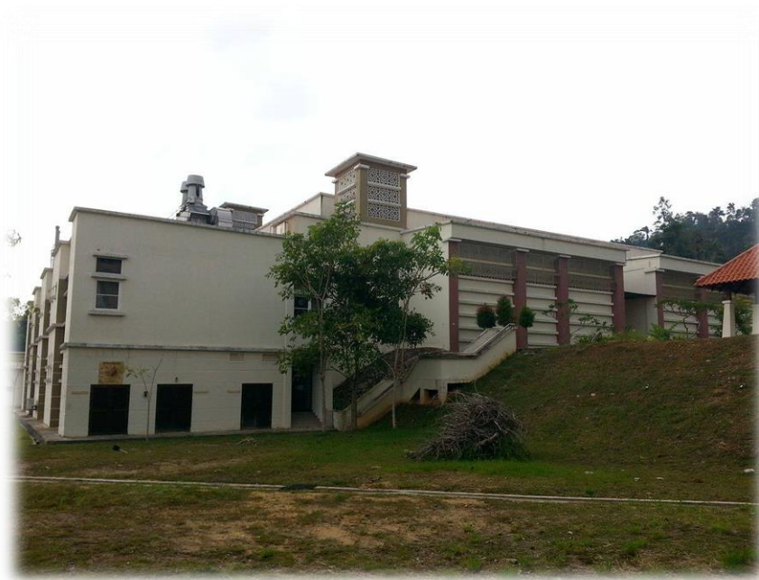
Figure 3.7 Side View (Right Elevation) of the Building (Middle of Slope)
