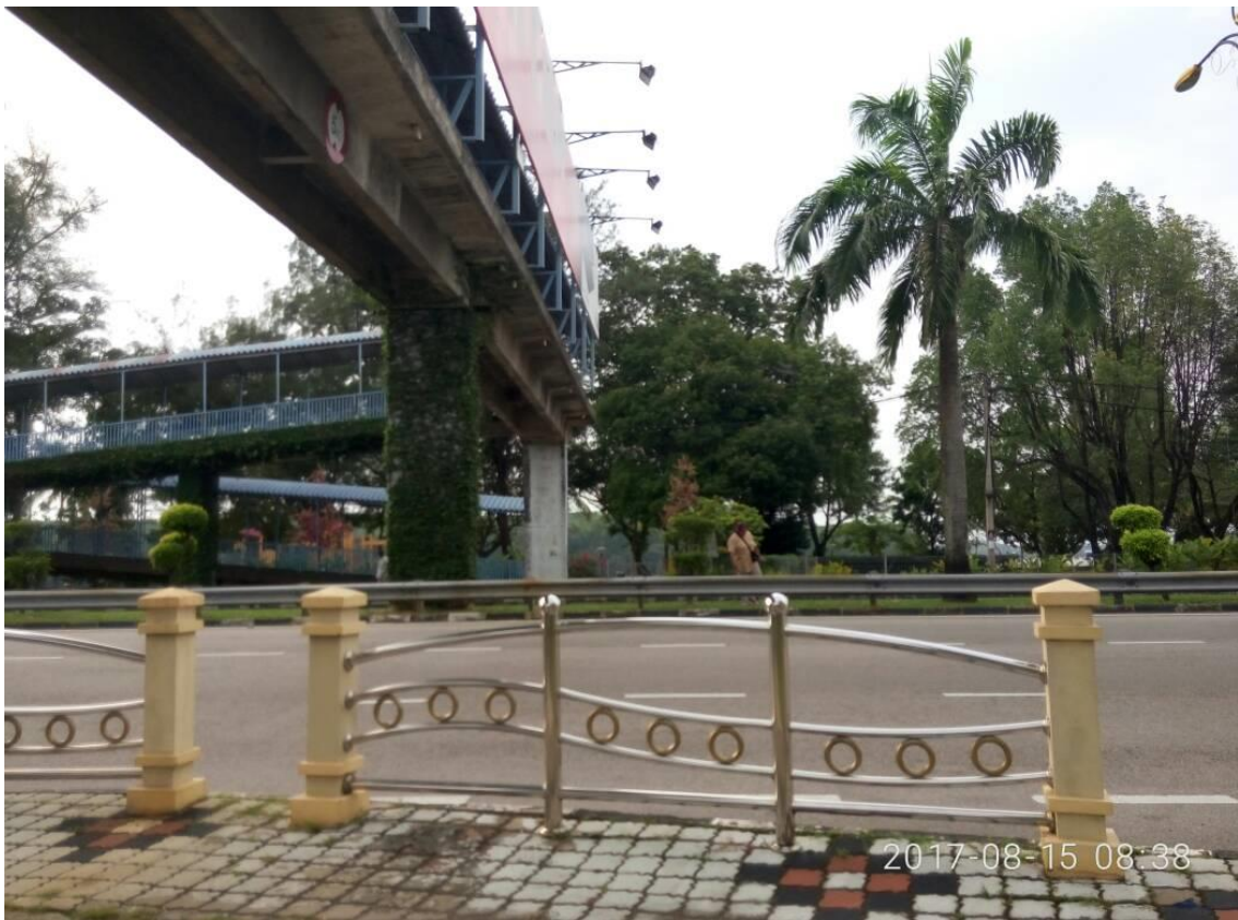
Figure 3-2: Pedestrian Bridge in front HTAA
