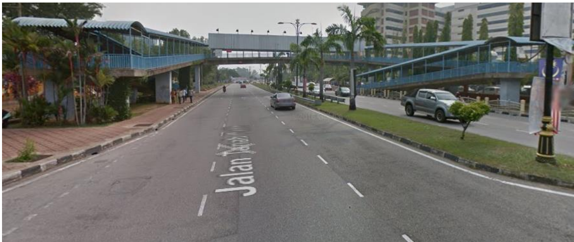
Figure 1-1: Pedestrian bridge at Jln Tanah Putih
